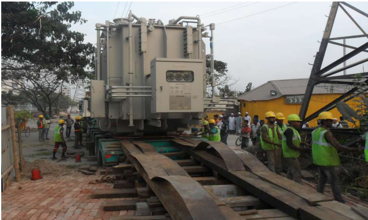
Picture 10 : Heavy cargo unloading from barge.
