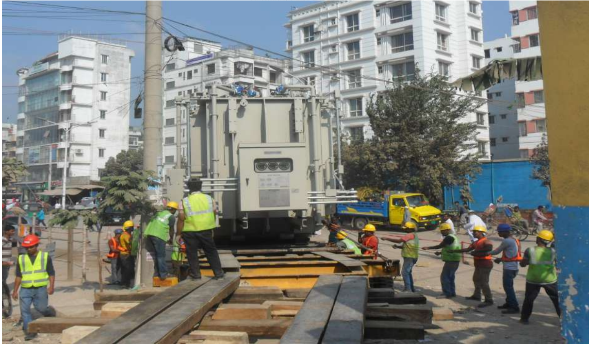
Picture 09 : Heavy cargo unloading from barge.
