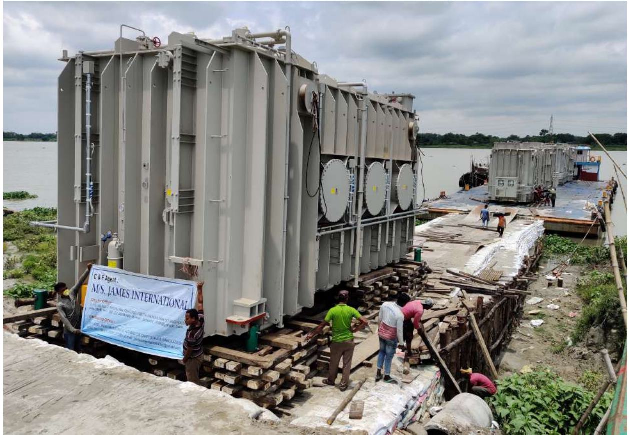
Picture 05 : Cargo discharging from Barge using Temporary.
