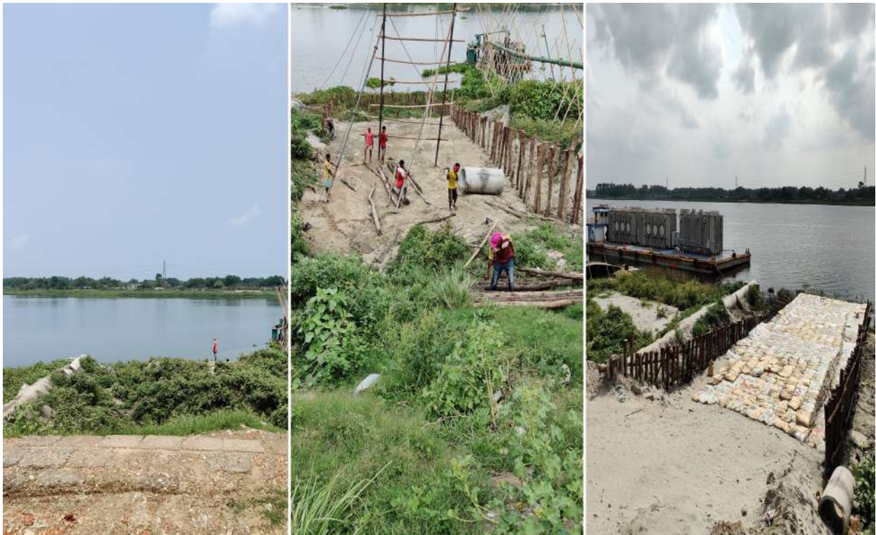
Picture 04 : Temporary jetty preparation to unload heavy cargo from barge.
